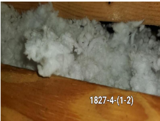
1827-4 Insulation/White Typical Interior
