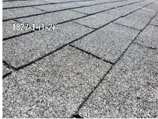
1827-1 Asphalt Shingle/Black Typical Exterior Roof
